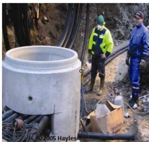
Figure 8. Installation of landfill gas collection lines at Rusko landfill (Hayles 2005).
