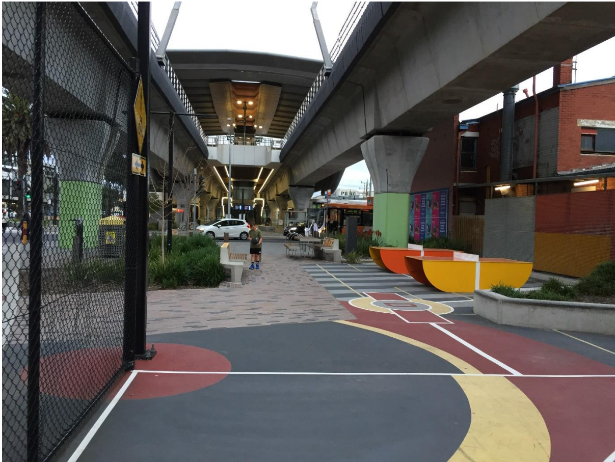
Figure 11- 4 Photograph of space below the Carnegie Station Skyrail area (Source: Walker, 2022)
