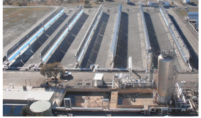
Fig. 1. Top view of the TCP-100 field at Plataforma Solar de Almería (PSA-CIEMAT). The three loops are shown, with two PTCs in each of them, numbered from 1 (rightmost) to 6 (leftmost). The first loop is formed by the connected pair 1-2 (right loop), the second loop by 3-4 (center loop) and the third by 5-6 (left loop).
