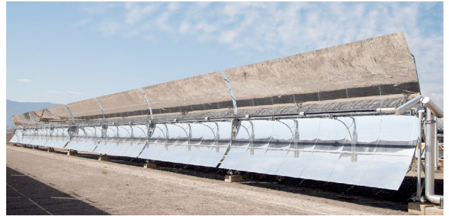
Fig. 2. Lateral view of the first PTC in the first loop at Pataforma Solar de Almería (PSA-CIEMAT). It is composed of 8 modules of 12 meters length.
