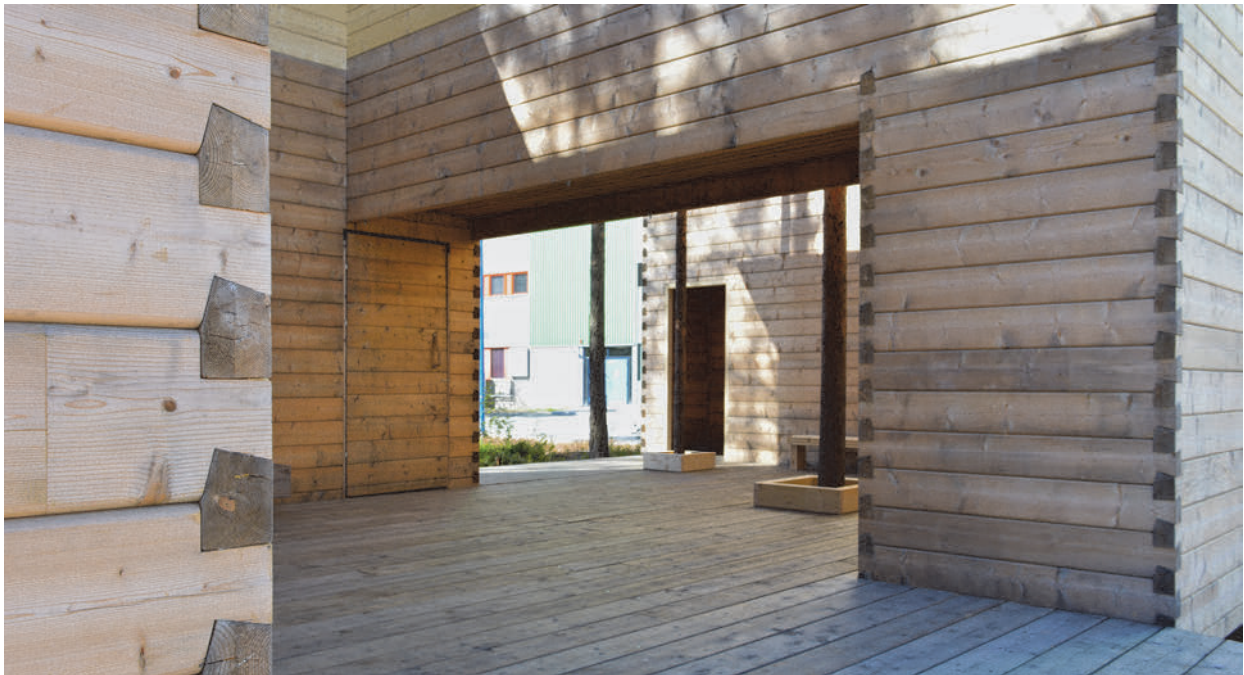
Fig. 8. The aspects of the Timber Tetris pavilion in Oulu brought up in this thematical category, such as the log construction method, corner joints and details of single logs are here well illustrated. Photo by the author.
