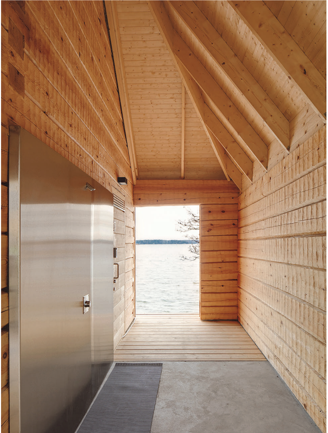
Fig. 24. The hand-hewn log surface in Lonna's sauna by OOPEAA Office for Peripheral Architecture. Photo: Jussi Tiainen. (Published with permission)
