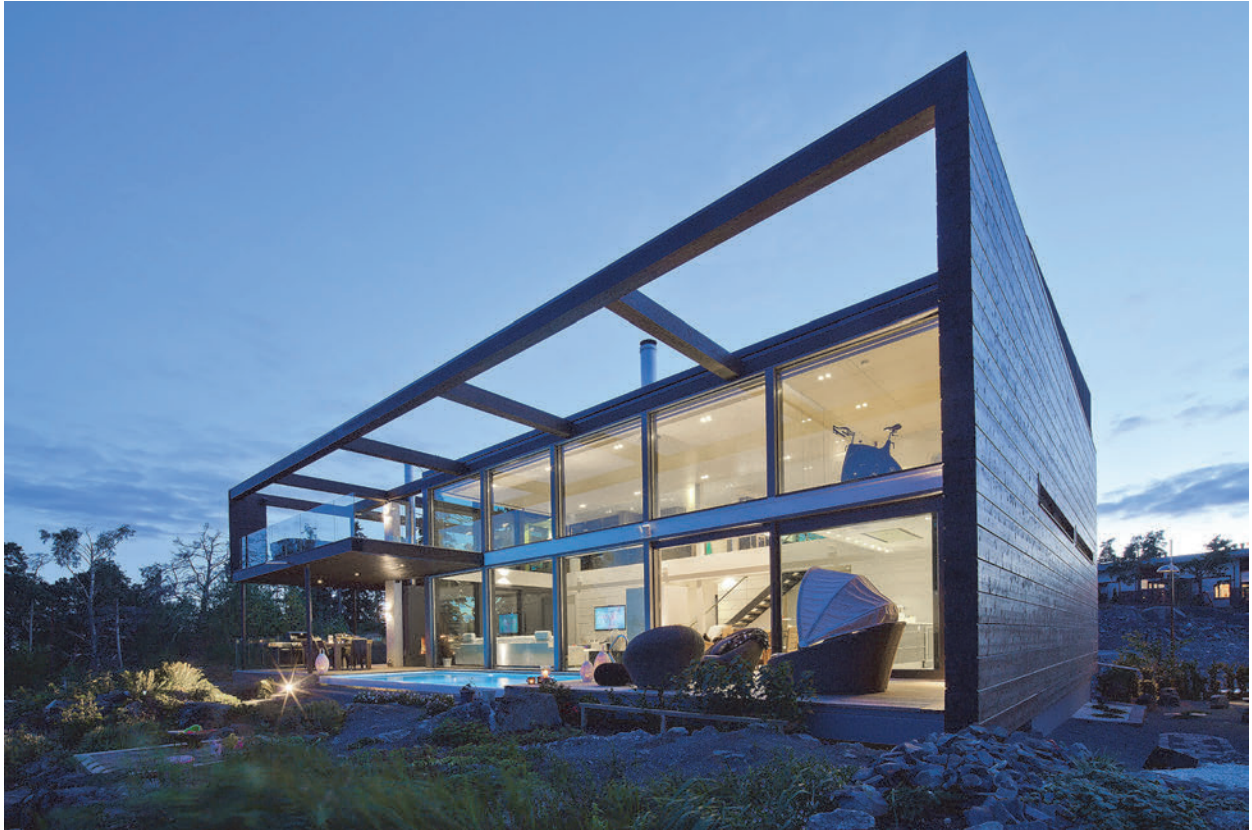
Fig. 19. Custom Home II (listed as building 1) by M.A.R.K. Architect's office Mäntylä, utilizes non-settling logs, to which steel reinforcements can be integrated, according to the respondents. Photo: Honkatalot. (Published with permission)
