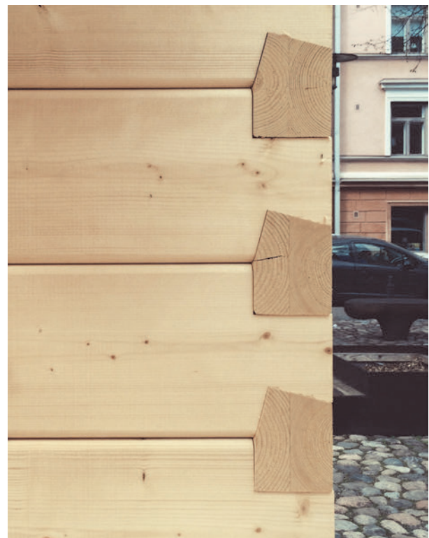
Fig. 9. Corner joints of the Timber Tetris pavilion in Helsinki. Photo: Aki Markkanen. (Published with permission)
