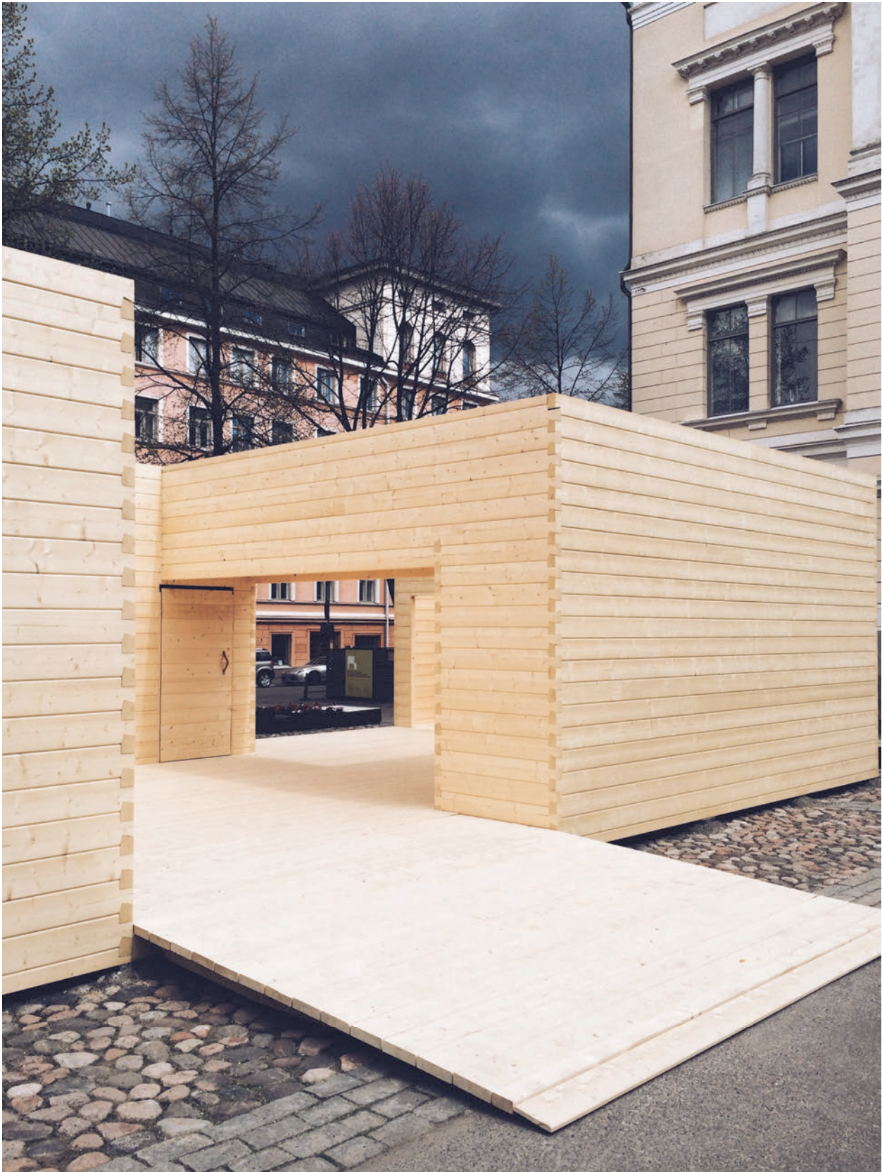
Fig. 2. The Timber Tetris pavilion in its original appearance in the urban milieu of Helsinki in 2017. Besides the horizontal lines between the logs, there are also some visible vertical seams within the logs, because of the finger joints that are used to lengthen the timber of the lamellas. Photo: Aki Markkanen. (Published with permission)
