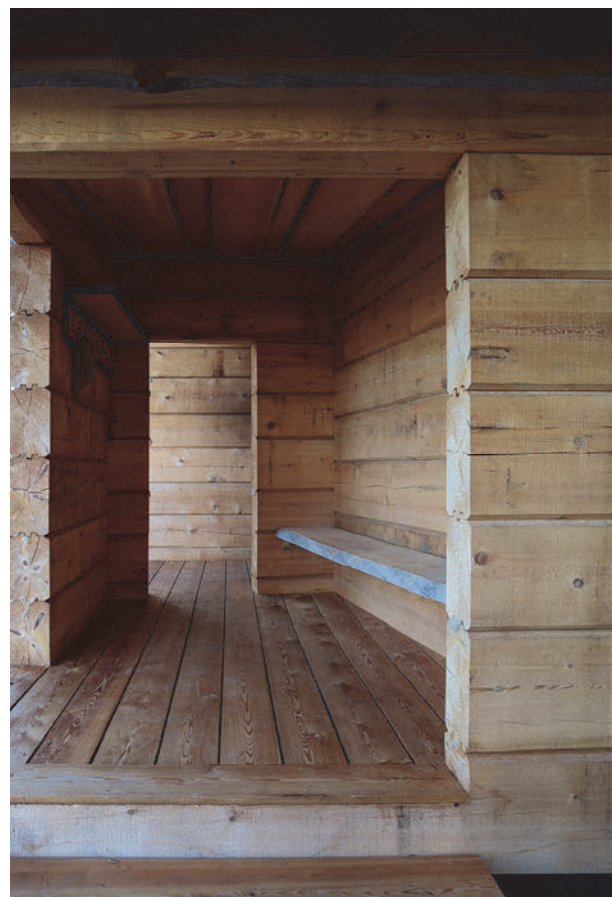
Fig. 15. Sauna Asikkala (listed as building 8) by Architect's office Tuomo Siitonen Ltd, utilizes non-glued sawn logs with industrially tooled tongues and grooves. Photo: Rauno Träskelin. (Published with permission)
