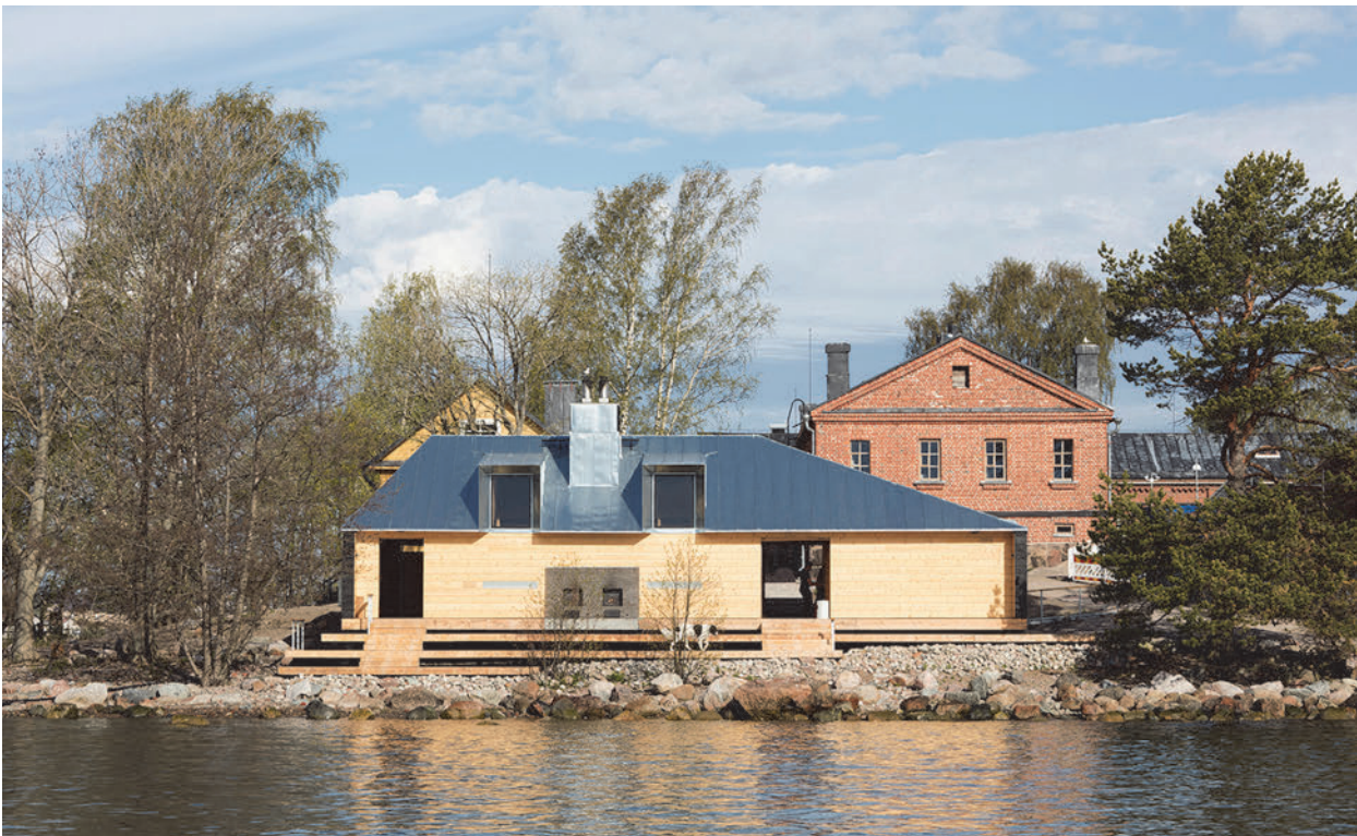
Fig. 20. The log structure of Lonna's sauna by OOPEAA Office for Peripheral Architecture is clad with a wooden board exterior. Photo: Jussi Tiainen. (Published with permission)
