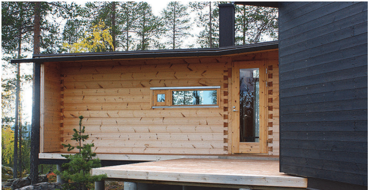
Fig. 21. In Villa Valtanen (listed as building 2) by Architect's office Louekari, the visible corner joints create ornamentation to the façades. Photo: Lauri Louekari. (Published with permission)
