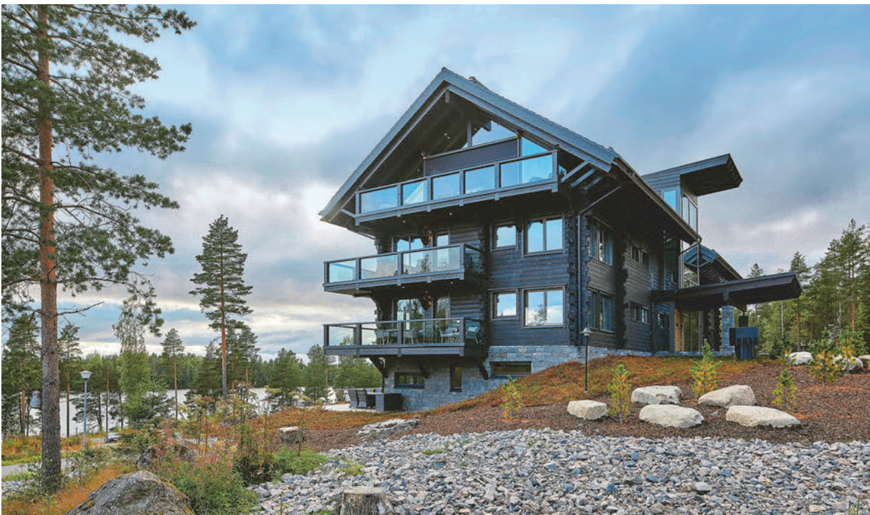
Fig. 22. Long corners are used in Naava Chalet (listed as building 6) by architect Janne Kantee in order to achieve the desired architectonic appearance seen fit for the surroundings by the corresponding architect. Photo: Honkatalot. (Published with permission)
