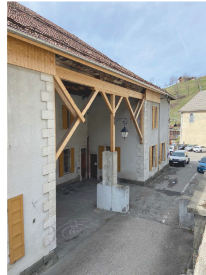
Fig.29 : The North East facade with the covered playground. We can still see on the ground the signs of children's games. We also see a new structure that takes up the weaknesses of the roof. © Angèle Golliet
