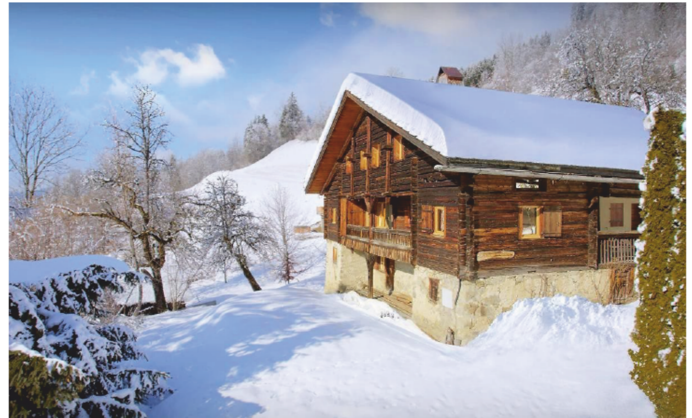
Fig.5 : Traditional house in Manigod with stone base and wooden elevation. We can see the three levels, the symmetrical facade, the small openings, and the large roof. The construction method of solid wood is also visible from the outside. We guess the different possible entries according to the slope. © Unknowned
