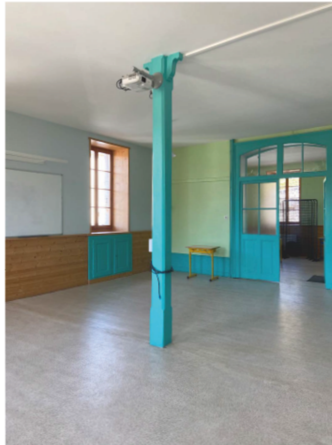
Fig.40 : One of the wooden columns that takes up the span.
