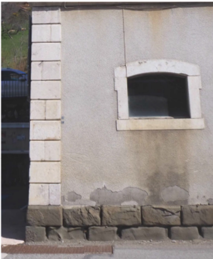
Fig.23 : The quoin and the stone base that anchors the building to the space. © Angèle Golliet
