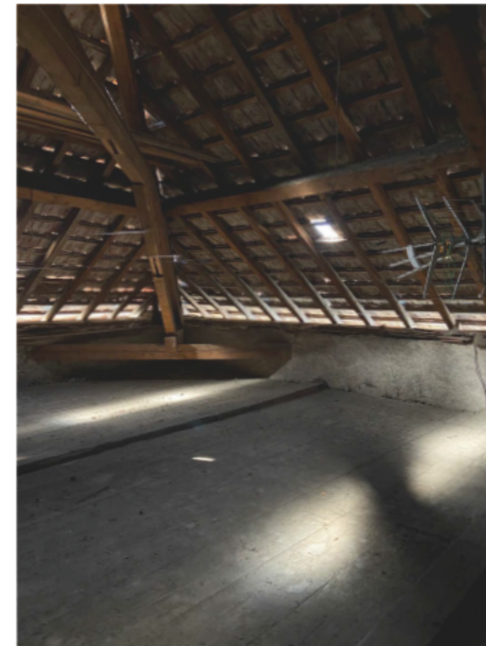
Fig.38 : The roof is only made of tiles, without insulation. Occasionally, there are transparent tiles that light up the attic. Here, the floor is a wooden one such as the two levels below.
