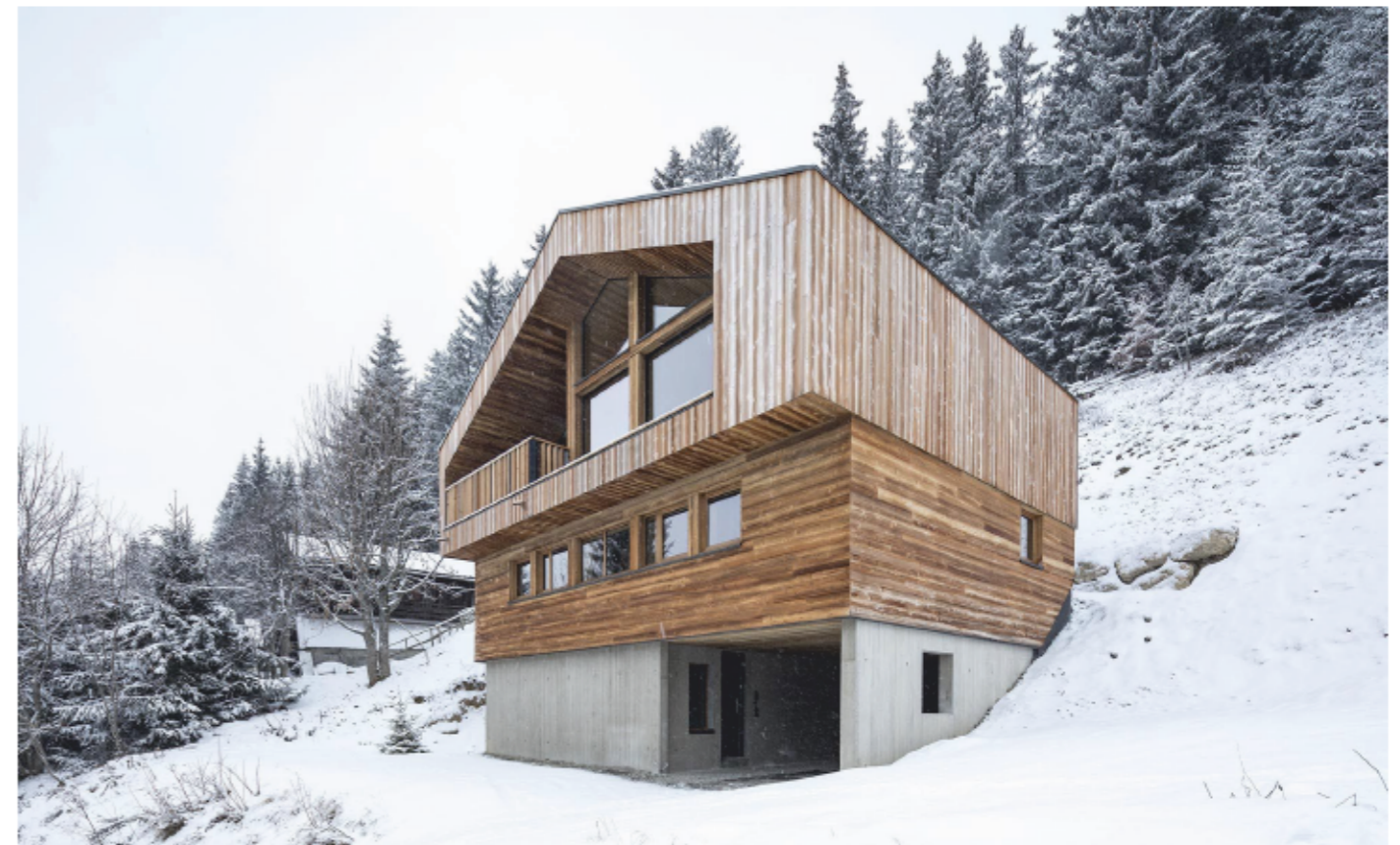
Fig.6 : Mountain House, a contemporary house by Studio Razavi Architecture in Manigod. The main differences are the concrete base, the roof aligned with the facade, and the large openings. The construction method and the number of floors are not perceptible. The entry seems only possible from the ground floor. © Studio Razavi Architecture
