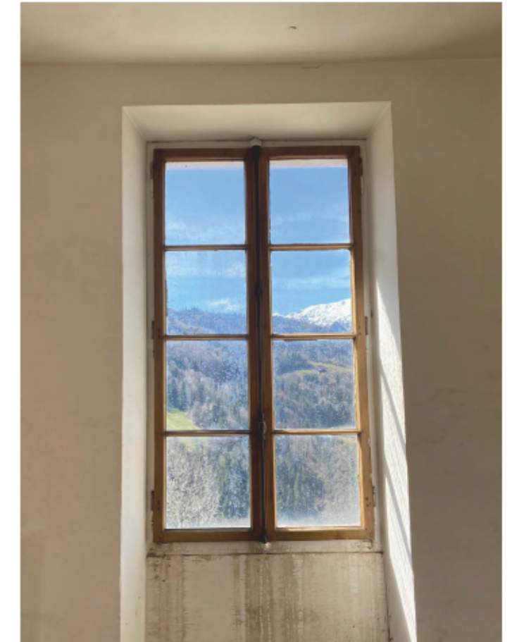
Fig.35 : There is a nice potential for natural light thanks to the existing large windows. Mark of humidity are visible on the walls near the window. This can be due to the simple glazed and the lack of insulation that does not help to maintain a comfortable space.
