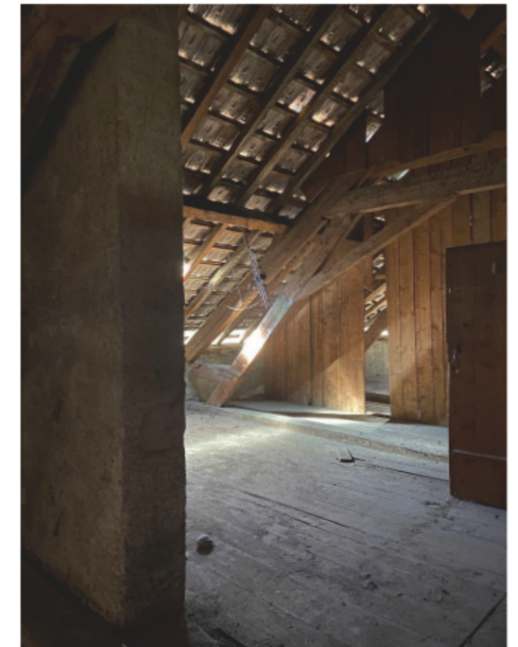
Fig.38 : The roof is only made of tiles, without insulation. Occasionally, there are transparent tiles that light up the attic. Here, the floor is a wooden one such as the two levels below.
