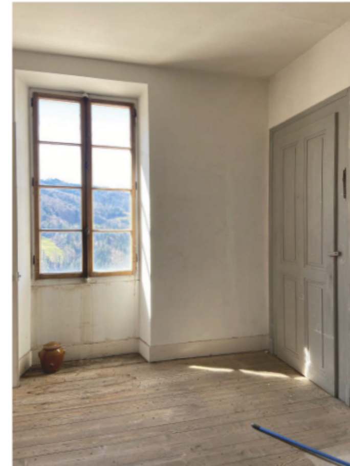
Fig.35 : There is a nice potential for natural light thanks to the existing large windows. Mark of humidity are visible on the walls near the window. This can be due to the simple glazed and the lack of insulation that does not help to maintain a comfortable space.
