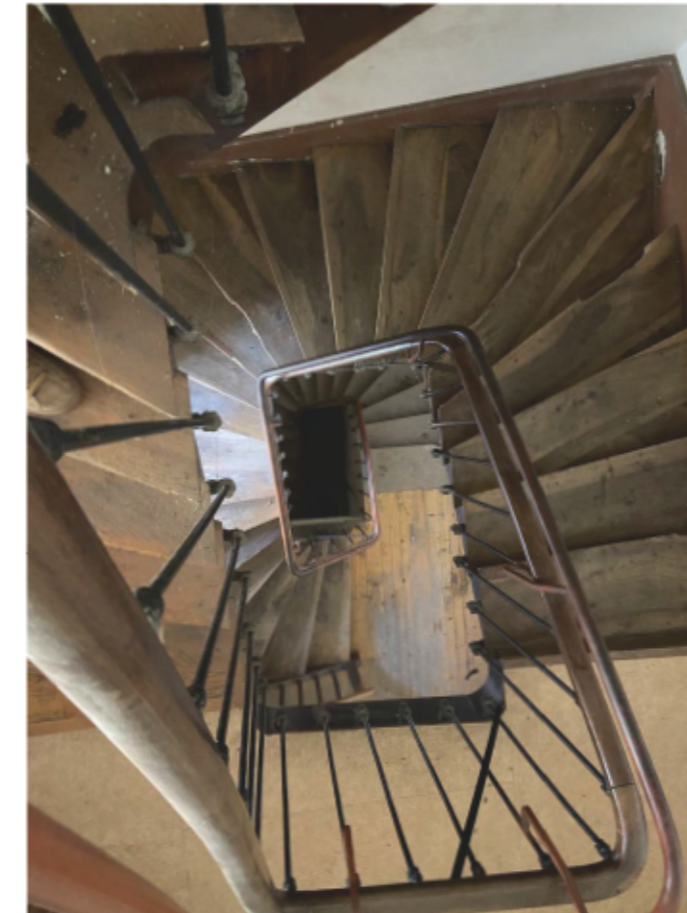
Fig.42 : The two wooden staircases crossing all the floors are not in good condition and need to be changed.
