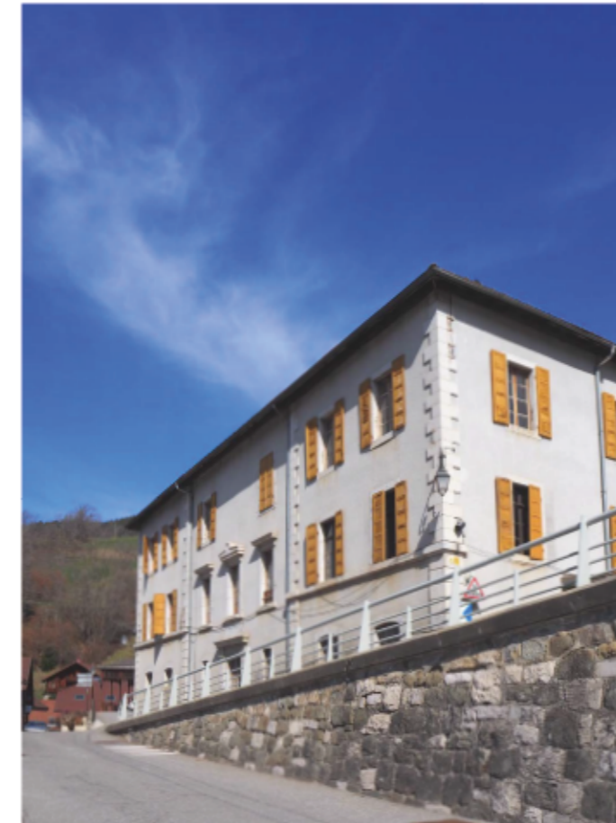
Fig.18 : The traditional main facade along the road D6 with the old main entry. © Angèle Golliet
