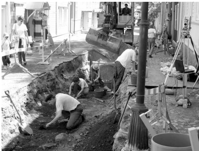
Fig. 2. Urban archaeology on Mannerheiminkatu street in the summer of 2002. Archaeologists with total stations and other equipment, a digger, as well as men from municipal engineering with water and sewage pipes are present on the site. The research only covered the area needed for installing the water and sewage pipes, the trench being c. 80 m long and 1.5-2 m wide.
