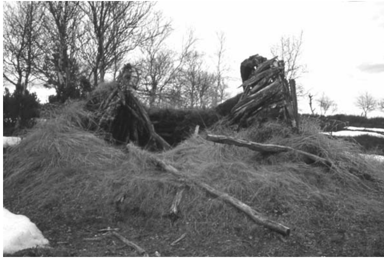
Fig. 9. Remains of a Saami turf hut in the Báišduottar – Paistunturi wilderness area, Utsjoki, Finland. The roof and parts of the walls have fallen in bringing inside the hut artefacts and structural parts that originally were outside. (Photo: T. Valtonen)
