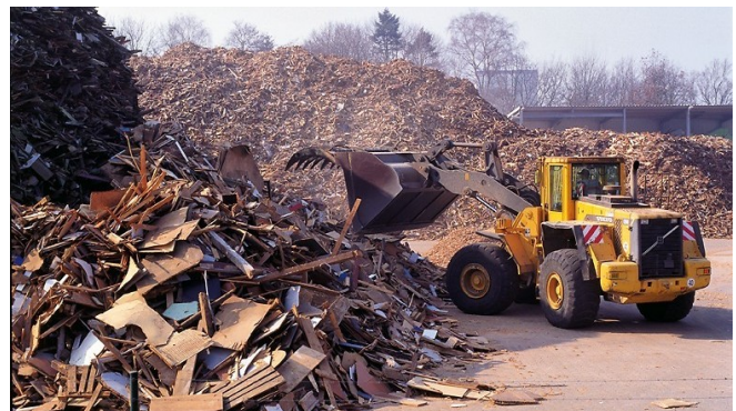
Fig. 2. Front-end loader and demolition wood [1].
