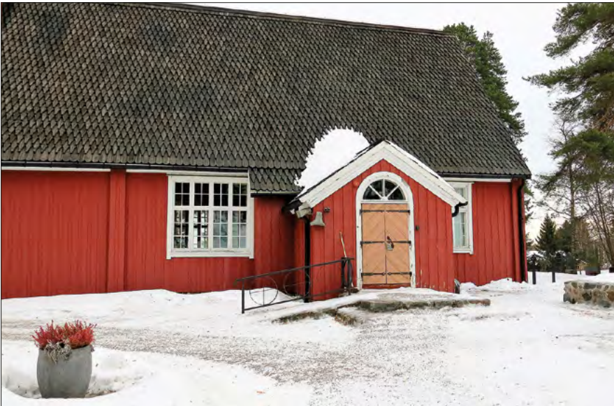
Fig. 2. The old wooden church of Kempele dates to the last decade of the 17 th century. It is currently under renovation that will take the preservation of the burials as well as the structures of the church into consideration. (photograph by Titta Kallio-Seppä).
