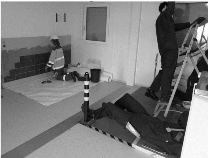
Fig. 2. An example of a training point focusing on construction work for house technology. The right side of the picture demonstrates problems related to bad planning (various different work phases performed simultaneously vs. scheduled work phases (left side))
