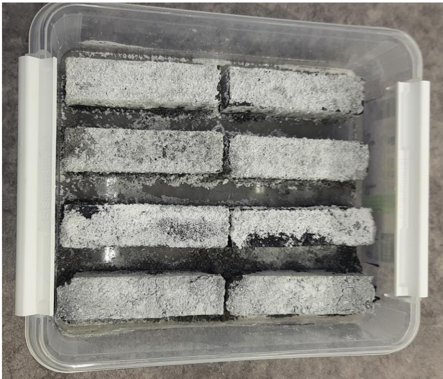
Figure 17. Efflorescence of the samples during the freeze-thaw experiments after 22 freeze-thaw cycles.
